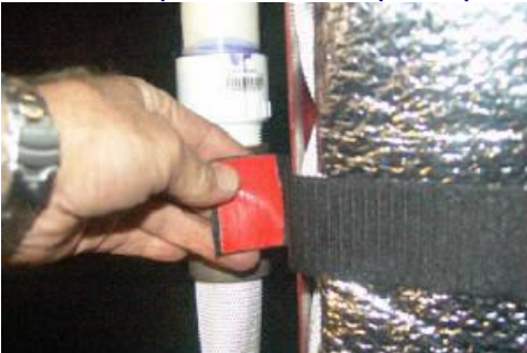
This strap secures the FIRE BLANKET and hose bundle in the cabinet box.
